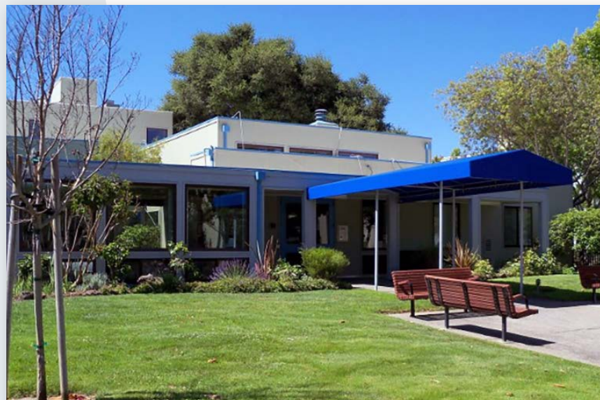
Property: Apartment complex with 101 one-bedroom units built in 1979 in PG&E service territory
