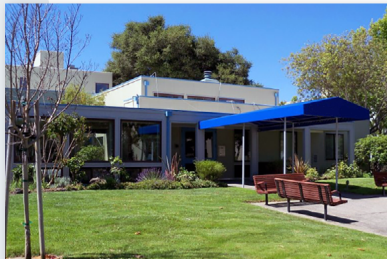
St. Mary's Gardens: Apartment complex with 101 one-bedroom units built in 1979 in PG&E service territory
