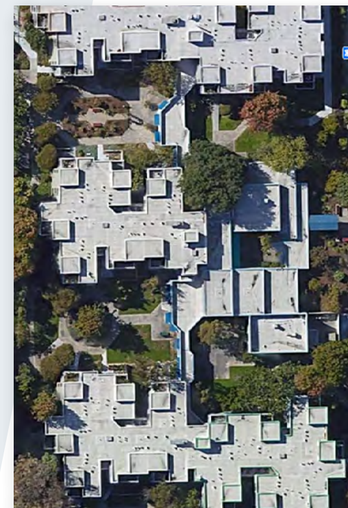
Location: Pacific Gas and Electric (PG&E) Service Territory Built: 1979 Units: 101 one-bedrooms
